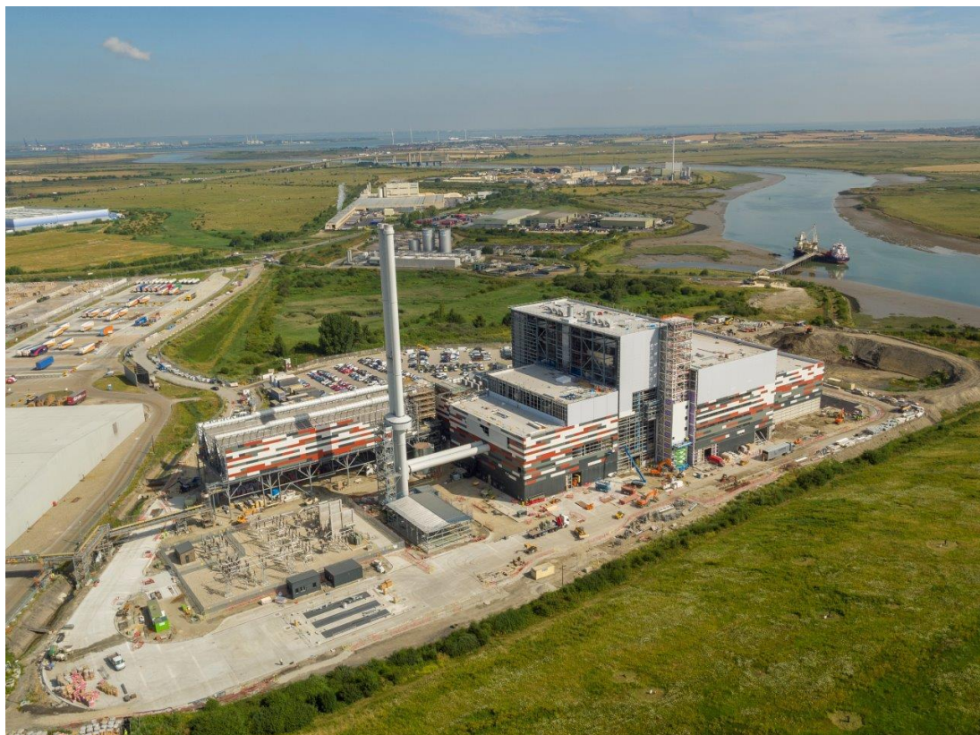
Figure 6.1 – K3 construction progress at July 2019.
